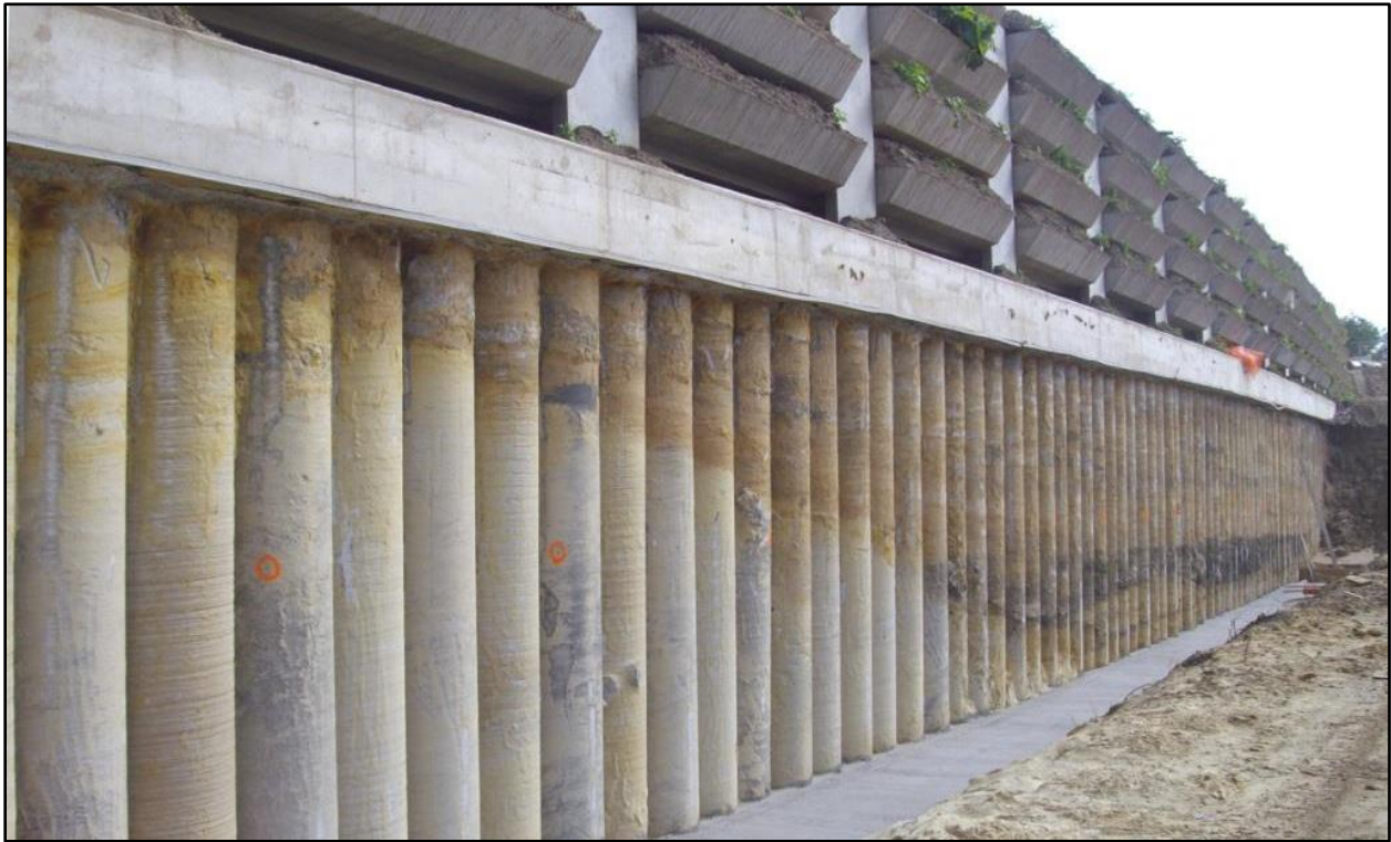
Figure 3-7. Typical Exposed Secant Pile Wall
