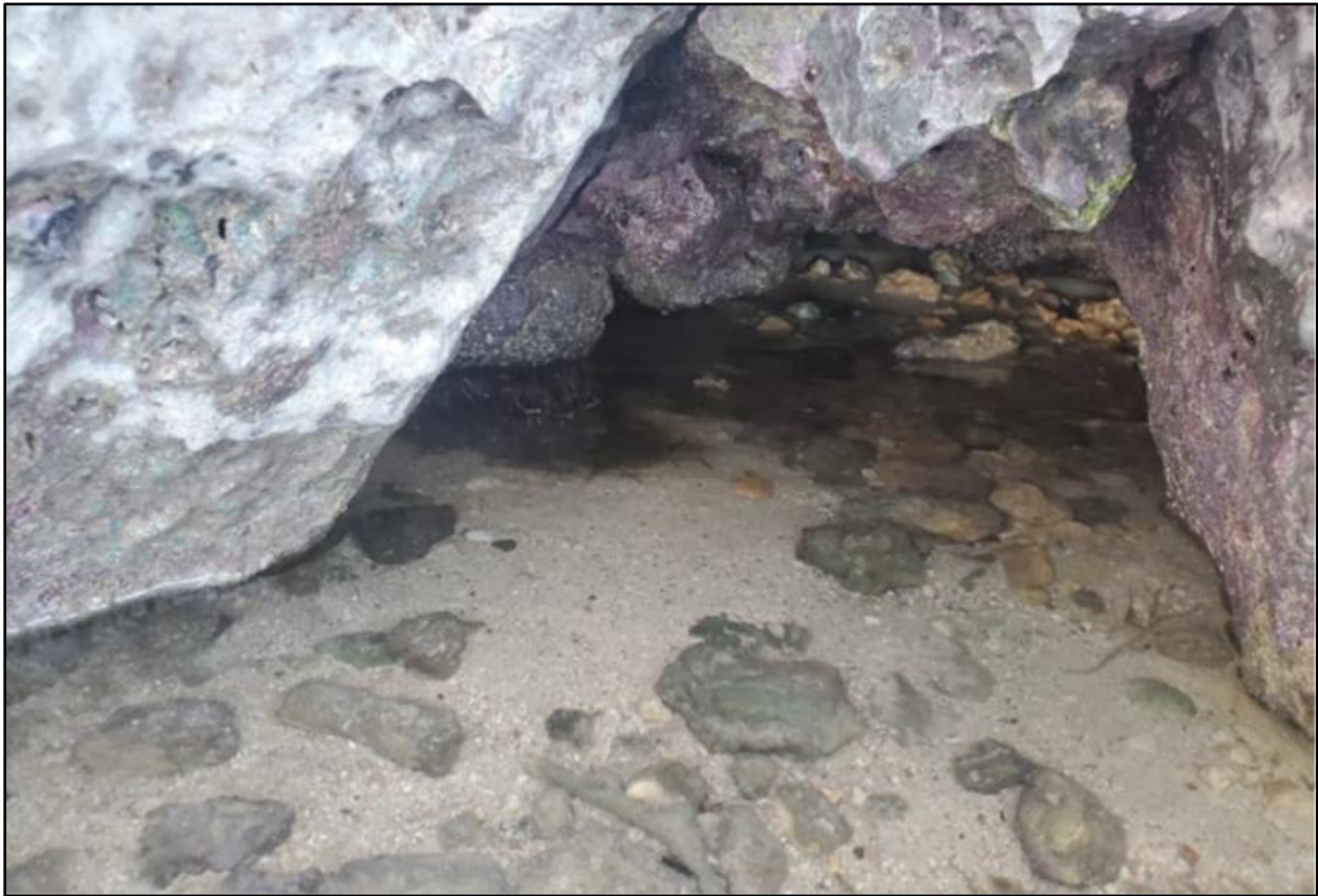
Figure 2-2. Undercutting of Existing Wall
