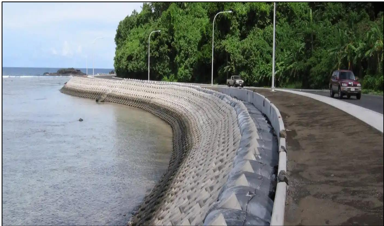
Figure 3-1. Typical Concrete Armor Unit (tribar) Revetment
