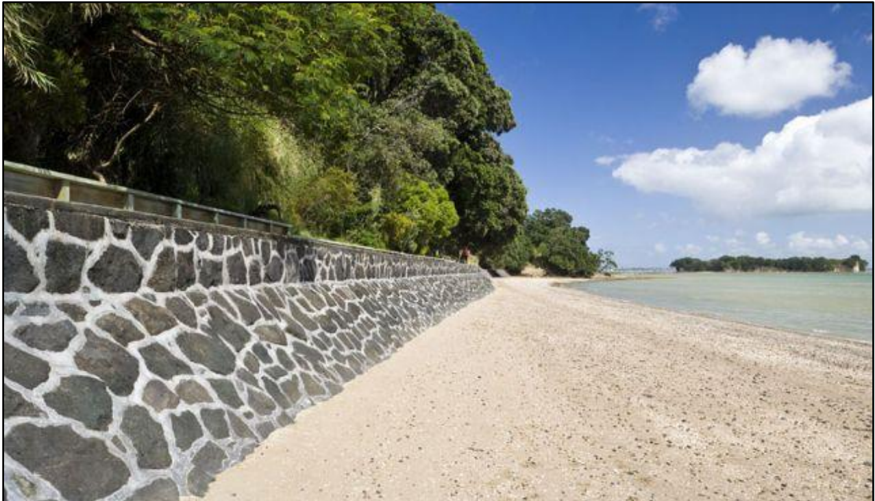
Figure 3-5. Typical surface of a Concrete Rubble Masonry Wall
